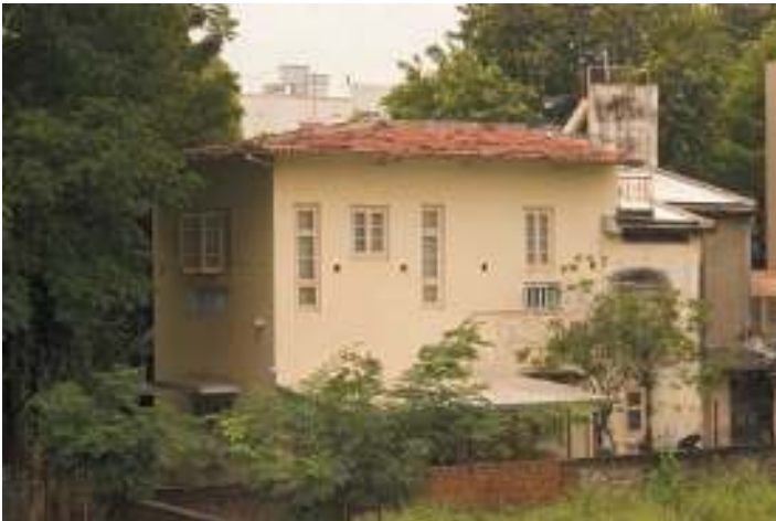
External view showing the small air inlets in the ventilated cavity wall, there are outlets at the upper level near the roof which are not visible
