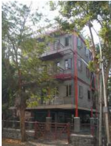
The completed structure
