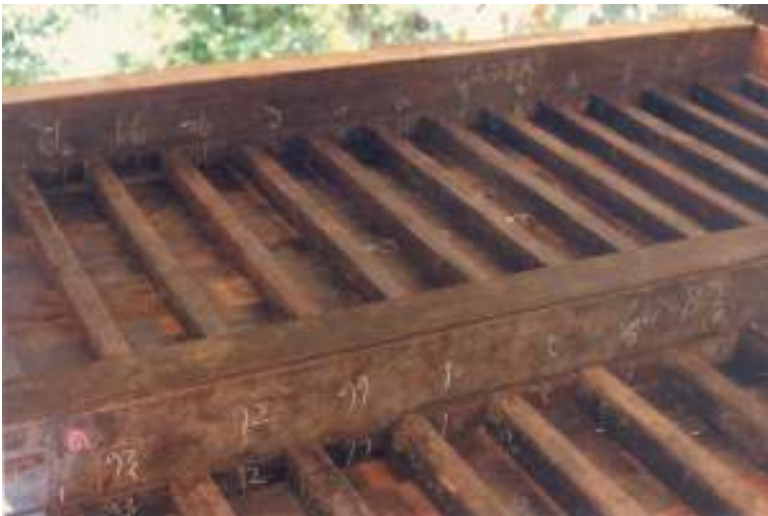
To ensure proper reassembling the wooden members were numbered before dismantling
