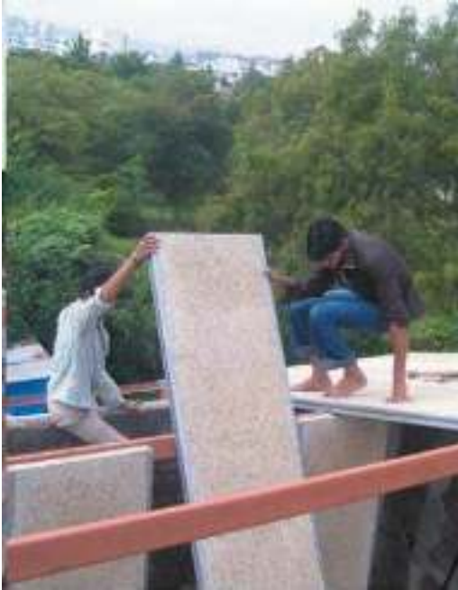
Wood wool board construction
