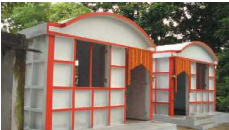
Completed one room kitchen house in ferrocement
