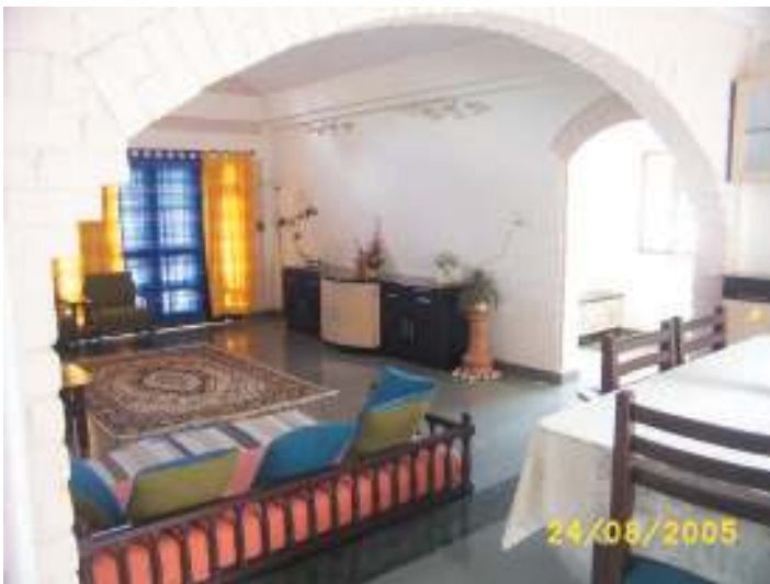
View of the interior. As structure is load bearing the arches are part of the structure.
