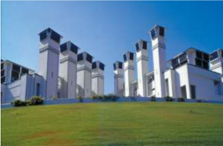
Torrent Research Centre : External view of the air exhaust shafts
