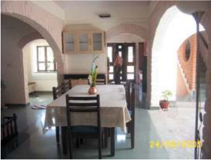
View of the interior. As structure is load bearing the arches are part of the structure.
