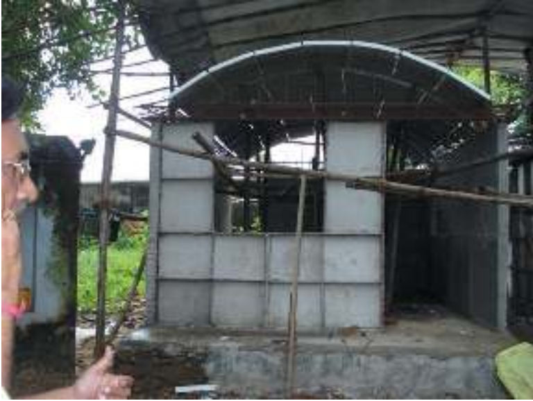
Precast ferrocement house – under construction
